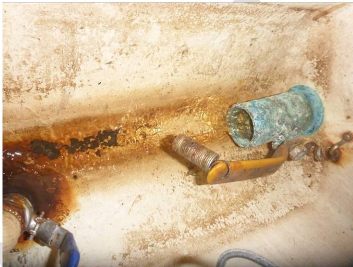
Forepeak valves should be swung regularly and checked for water.
